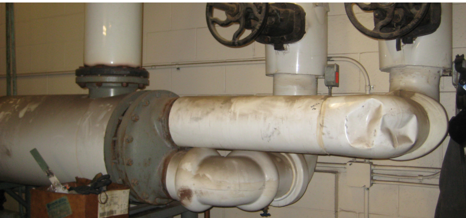
Figure 81 - Heat exchanger
