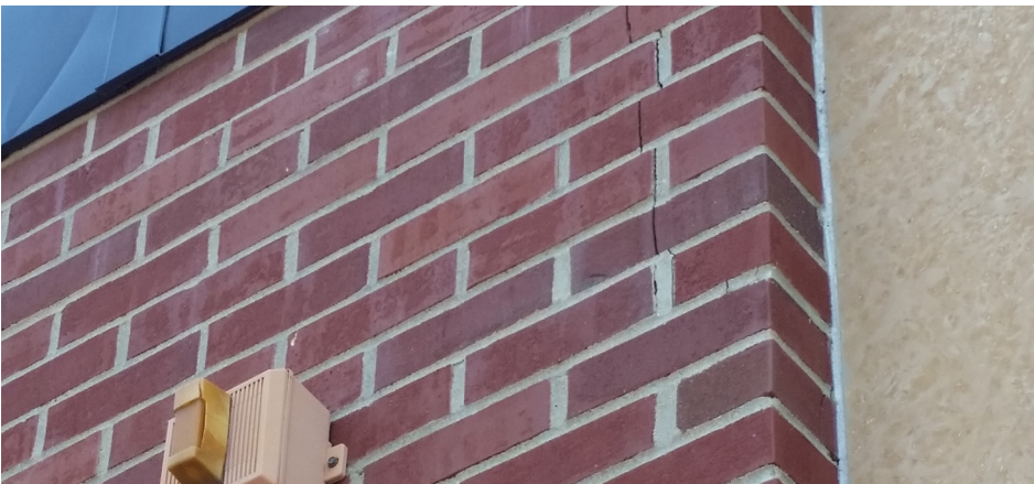
Figure 27 - Cracked brick location
