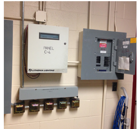
Figure 94 - Lighting control panel
