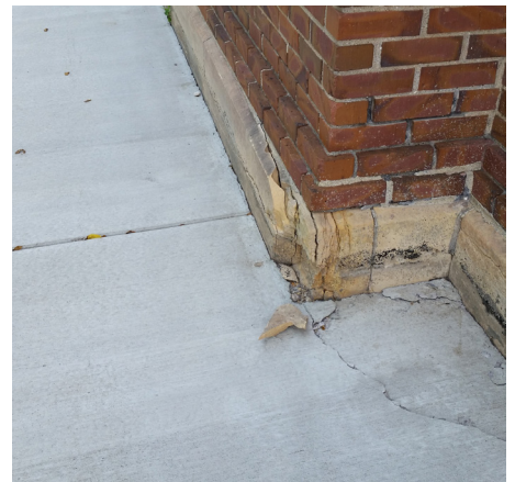
Figure 21 - Deteriorating exterior stone on west side near Gym
