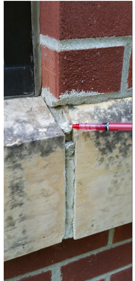
Figure 22 - Deteriorating grout
