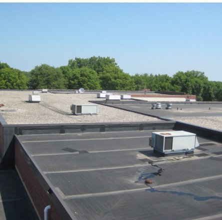
Figure 83 - Typical DX rooftop unit
