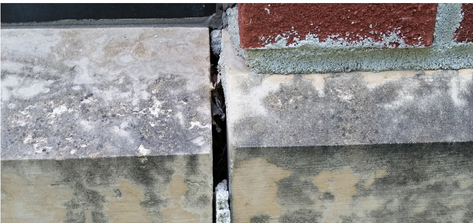
Figure 23 - Deteriorating grout
