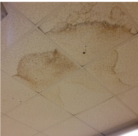
Figure 62 - Stained ceiling tiles
