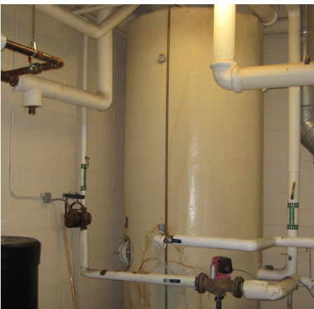
Figure 77 - Domestic hot water storage tank
