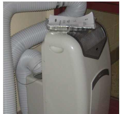
Figure 93 - Portable cooling unit
