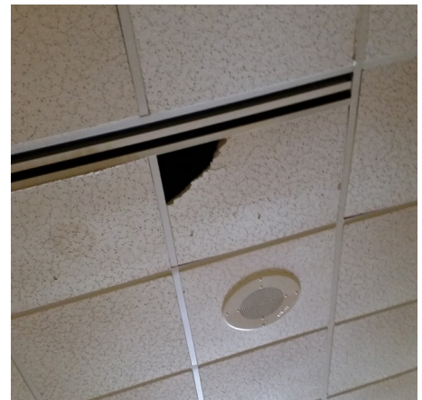
Figure 40 - Broken ceiling tile
