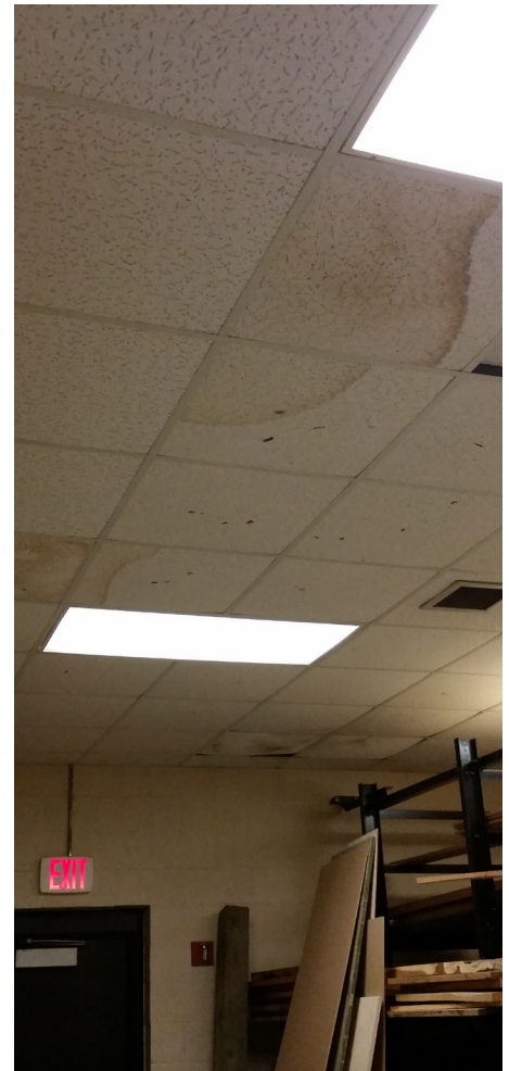
Figure 61 - Stained ceiling tiles
