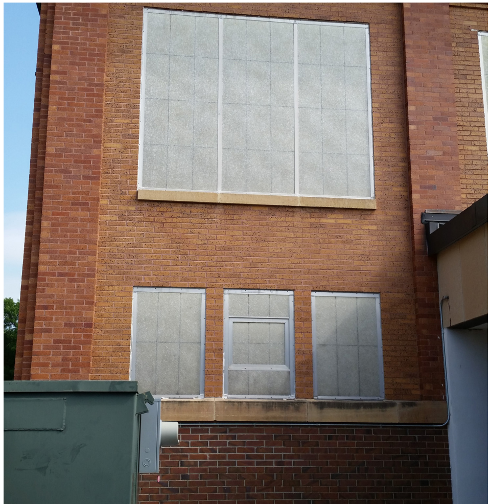
Figure 36 - Kalwall window type
