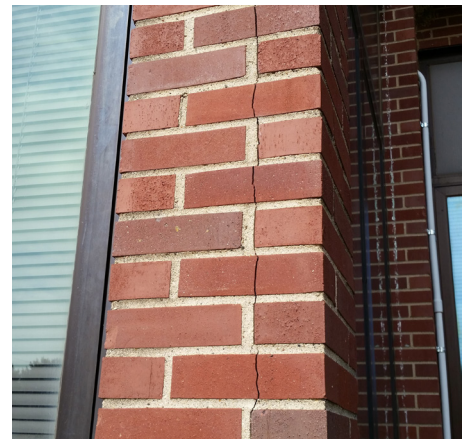
Figure 28 - Cracked brick location
