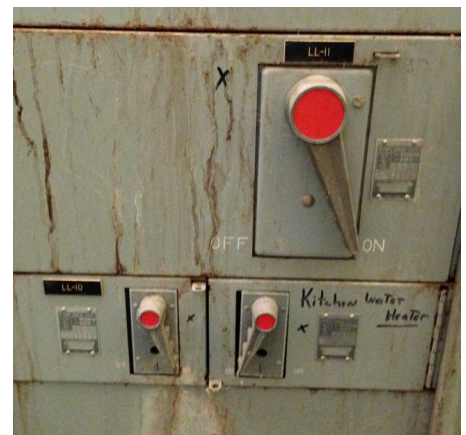
Figure 95 - Original electrical service with water stained cabinet
