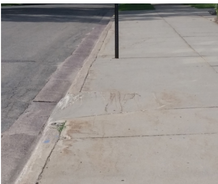
Figure 3 - East side sidewalk accessibility ramp
