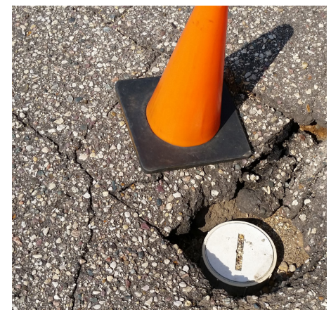
Figure 9 - Clean-out hole safety hazard in asphalt paving
