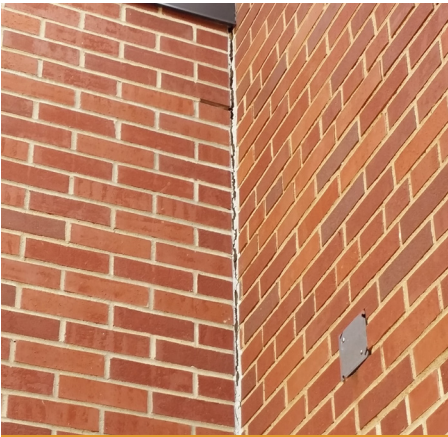
Figure 25 - Voids in exterior caulk joint
