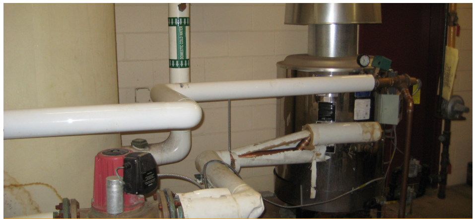
Figure 76 - Domestic hot water boiler
