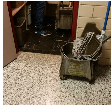
Figure 70 - 9x9 floor tile in janitor closet
