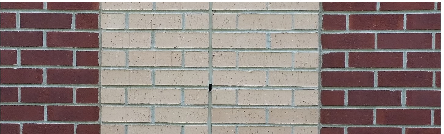
Figure 24 - Void in exterior caulk joint
